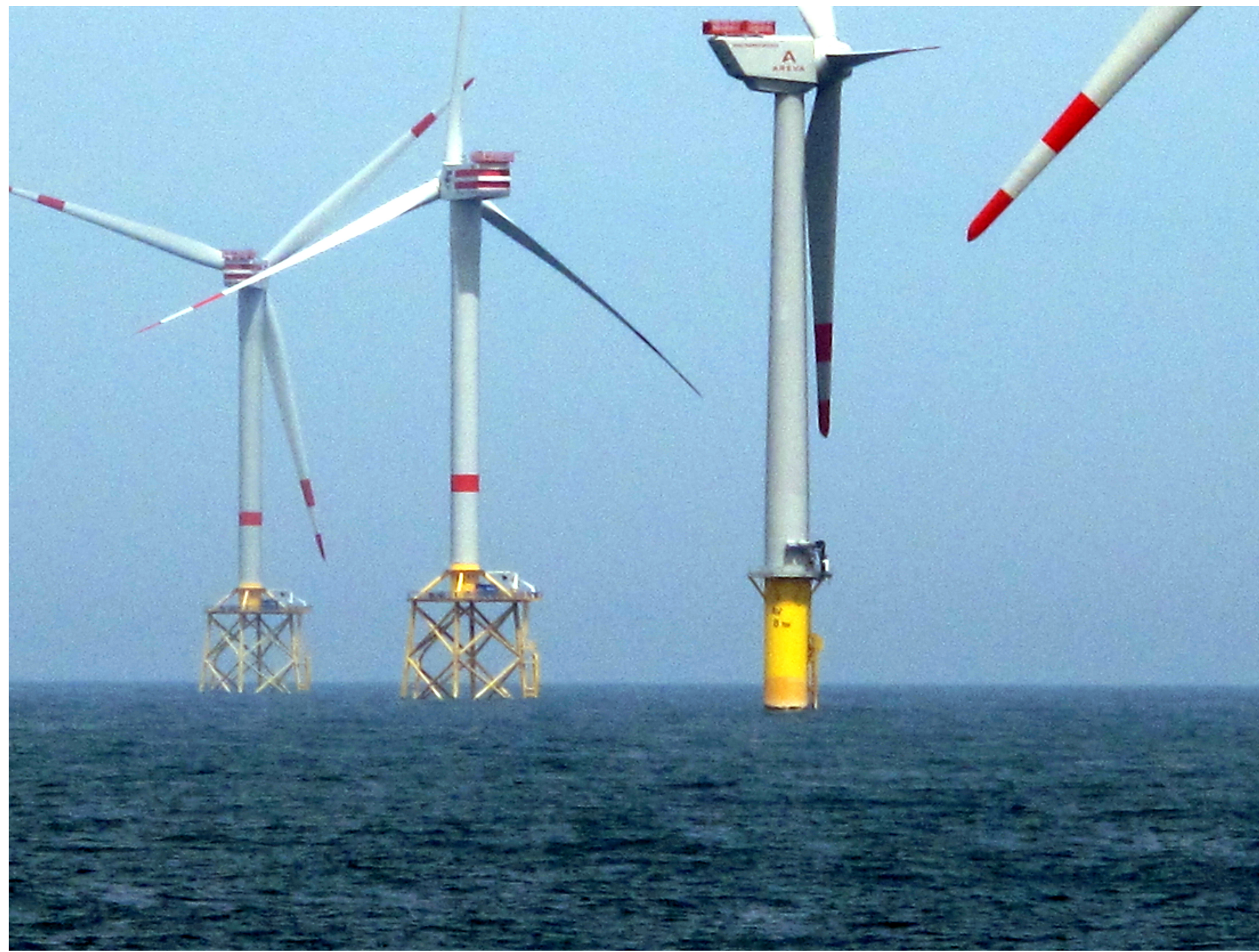
Fixed bottom offshore wind turbines on jacket structures (left two) and monopile (right turbine) from (1).
