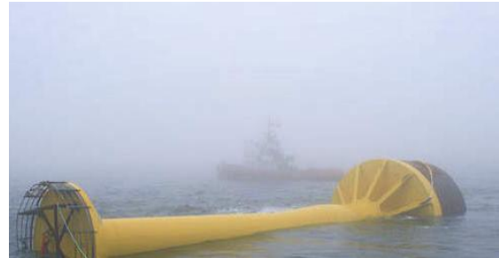
Figure 10: Float-out foundation (MBD Ocean Power)
